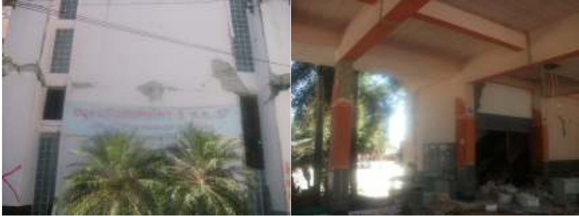
(a) Four stories school building
